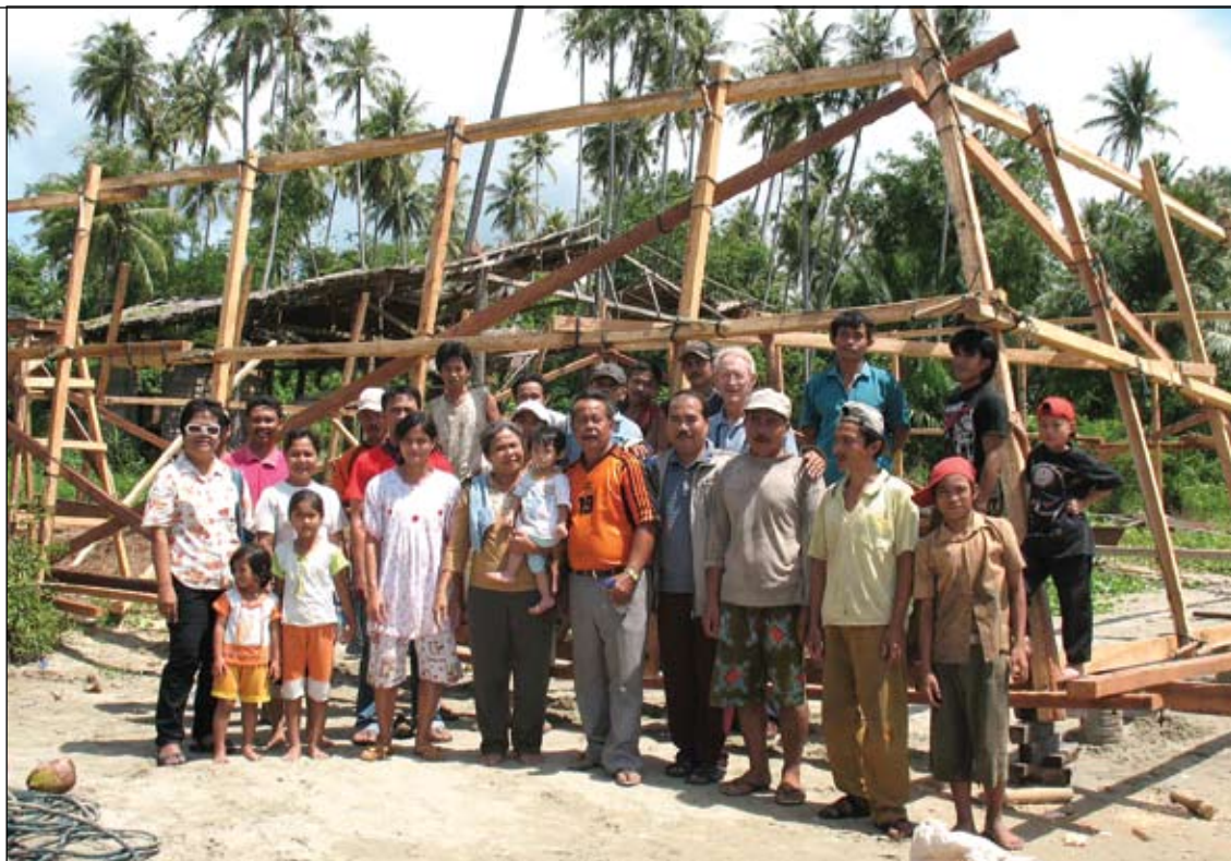
Villagers build a fishing platform that since completion has been moved out to sea.
